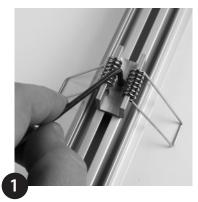
Cut a 30-32mm (1.2-1.26") wide slot to the required length. Bring through power feed and make connection.
